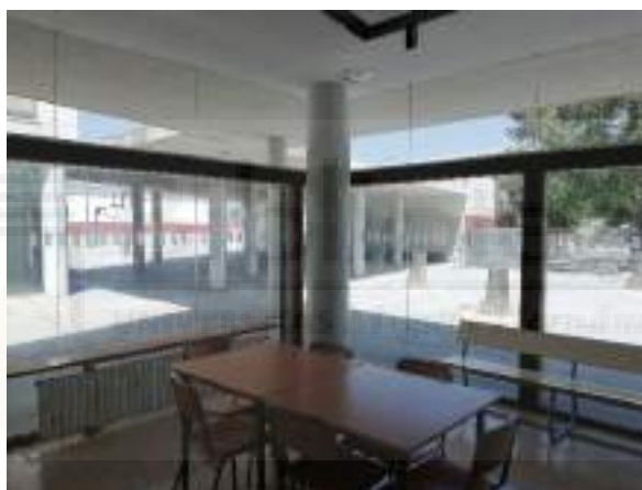
Figure 7. “Fish tank” cafeteria without natural ventilation in a modern school.
