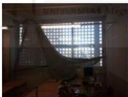
Figure 5. Oversize window and rolling blind, not easy to handle and more expensive for maintenance and repairs.
