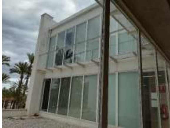
Figure 12. “Walk-out windows” seen from the outside.
